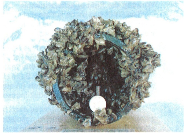
It took only three months for mussels to completely cover and block this once-clean pipe. One breeding pair of invasive mussels produces more than a million offspring each season.
